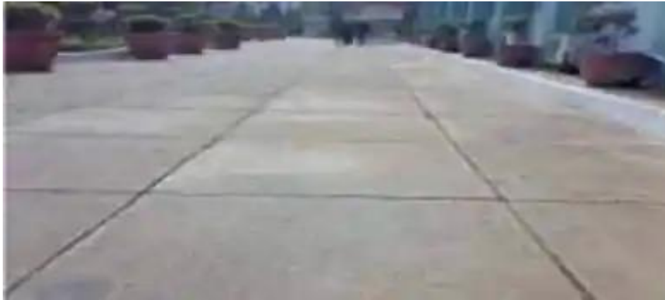
Figure 3-2: Pavement with steel fiber reinforced concrete
