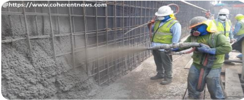
Figure 2-11: The process of pouring shotcrete for a concrete wall
