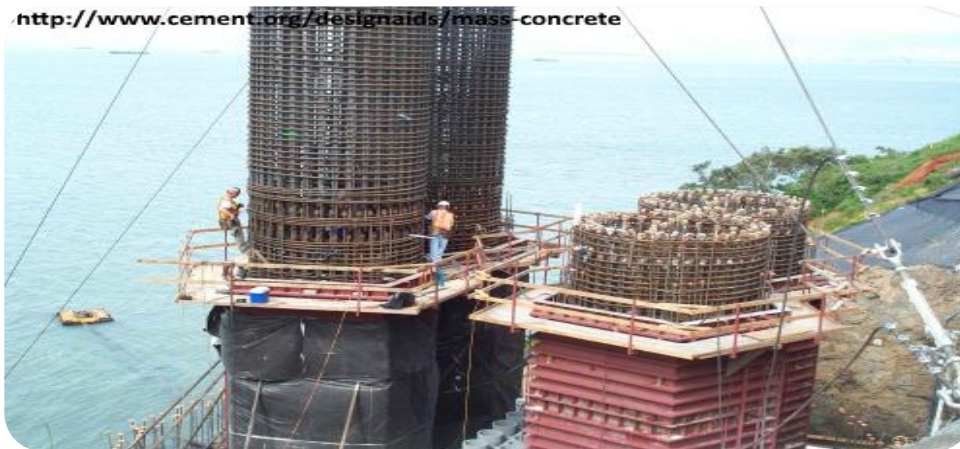
Figure 2-12 : Pouring large quantities of concrete in a bridge project
