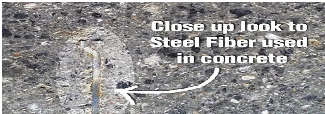
Figure 3-3: Steel Fibers in Concrete
