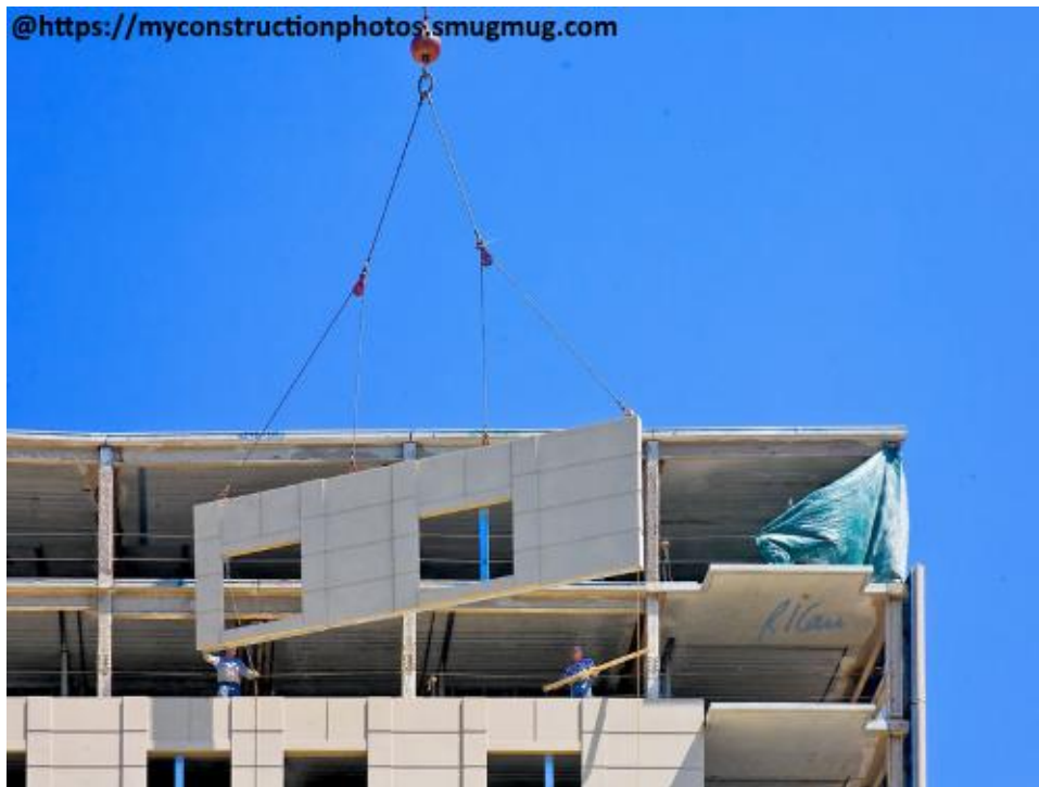
Figure 2-8: Installation of precast elements in a housing project
